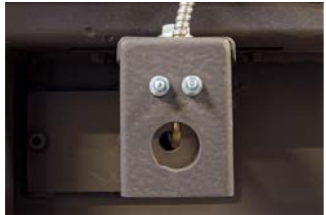
For filling level control, the light barrier had to be placed laterally, in contrast to the rotating paddle level detector, so that the fiber optic can detect the combustion chamber through a hole, as shown here. (Image: ipf electronic)
