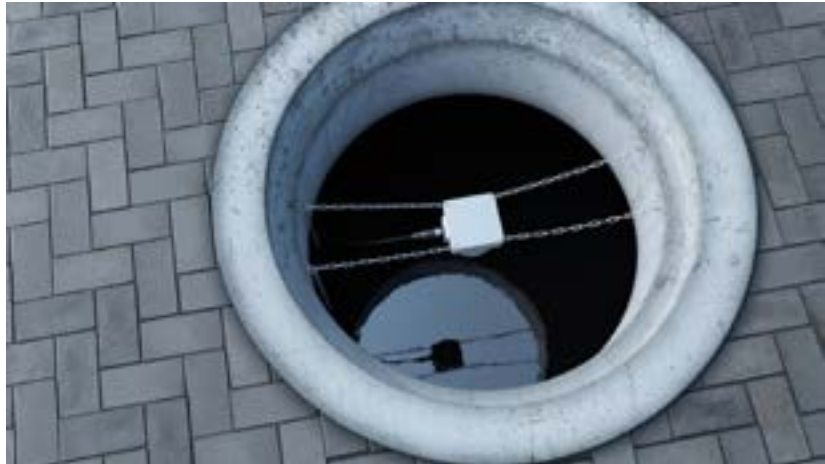
Fig. 18: A UT800320 ultrasonic sensor for sensing the water level in a cistern.
