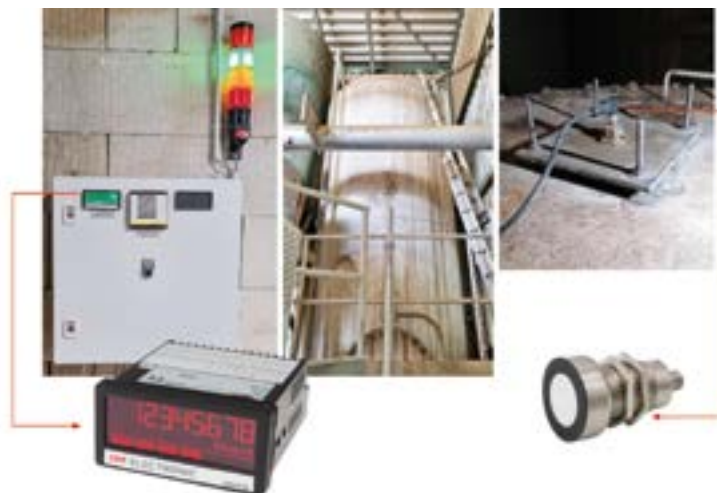
Fig. 29: The ultrasonic diffuse-reflection sensors were mounted in the lid area of a silo container (right). The transmitter (left)
