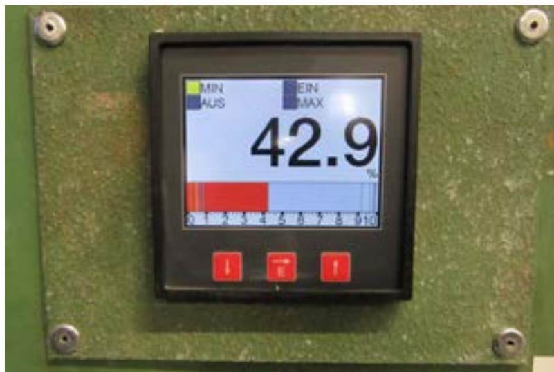
Fig. 35: The BA960900 digital transmitter processes the level sensor current signals preset for the maximum and minimum levels.
