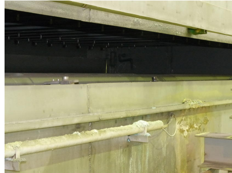
Three parallel-operated inductive sensors are positioned at the input and output of the pickling chamber. The special arrangement ensures that a larger area of the copper plate can be inquired from the underside and thus at least one sensor responds.
