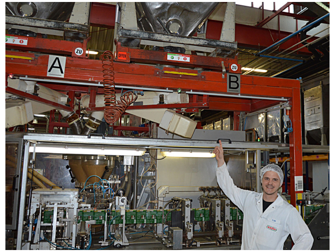
Rudolf Kau shows how the signal solution was integrated into the overall concept of the filling plant. The compact LED lights do not prevent the forklift truck from maneuvering and they cannot be damaged accidentally by a forklift truck's fork.
