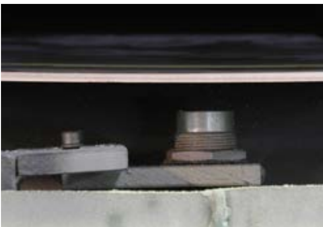
The inductive sensors IO300106 were installed in a way that they can detect the copper plates from below.
