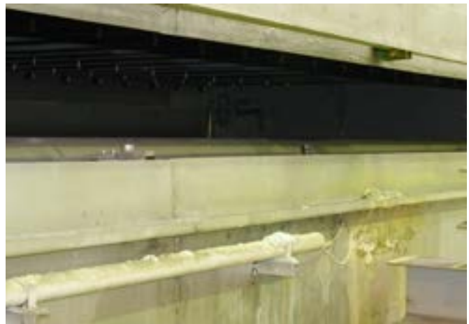
In each case three inductive sensors are positioned at the entrance and exit of the pickling chamber. The special arrangement ensures that a larger area of the copper plate can be queried from the underside and thus at least one sensor responds.
