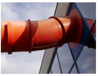
A high-performance light barriers is located underneath the cover (left) immediately behind the entrance to the slide.
