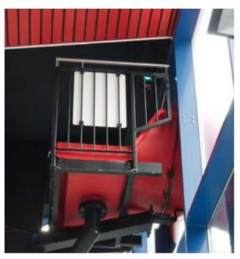
The traffic lights in the indoor pool are controlled by a PLC connected to the amplifiers of the high-performance light barriers.
