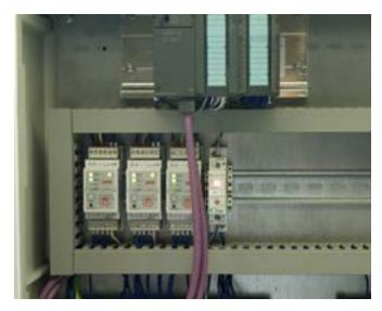
The space-saving mounting of the single-channel amplifier **OV620810** with switching and analog output on a top-hat rail in the control cabinet below the PLC.
