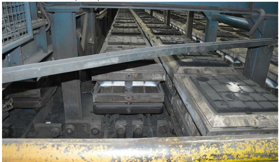
Inductive sensors and conventional optical scanners repeatedly led to problems in the container station.
